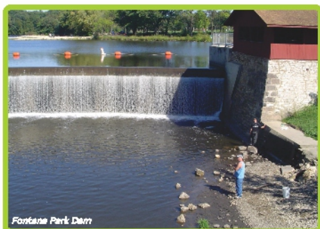
Fontana Park Dam
